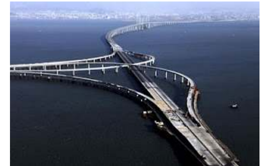
Puente Qingdao Haiwan (42.5km)
