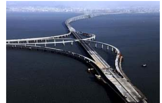
Puente Qingdao Haiwan (42.5km)
